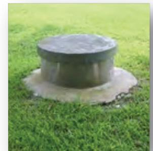
*[right] Bored well [top] and drilled well [bottom] with proper casing and secure well cap*
