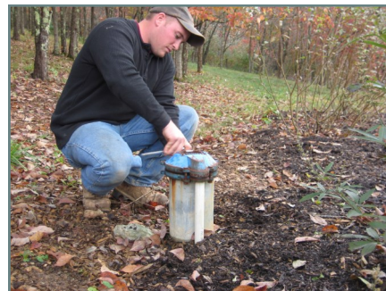
A professional well drilling contractor opening the well cap for shock chlorination.
